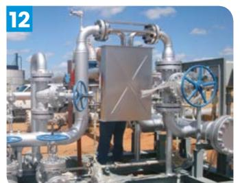
13. OILFIELD SERVICES Rheonik high pressure meters provide close-to-the-well flow measurement with high turndown capability and fluid independence for the utmost in deployment flexibility
